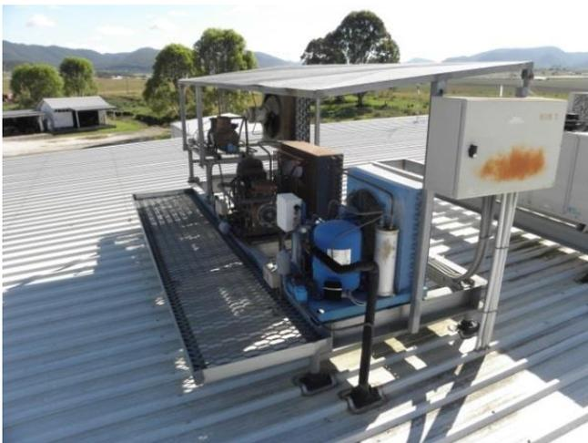
Position the condensing unit or air cooled condenser clear of the ground and on the roof.
