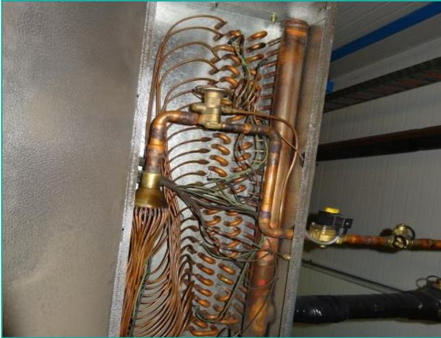
Install solenoid valve close the expansion valve
