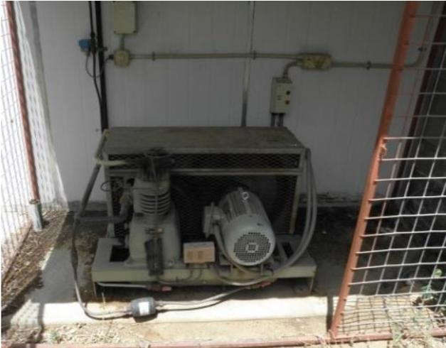
Avoid enclosing and placing on the ground.
