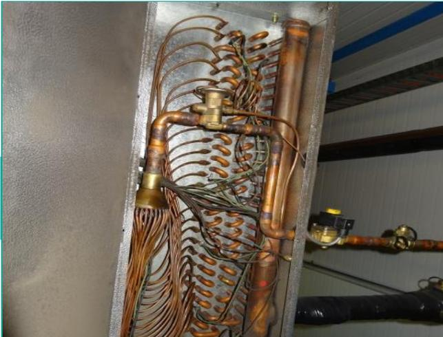
Install solenoid valve close the expansion valve
