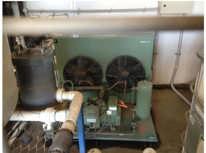
Install solenoid valve close the expansion valve
